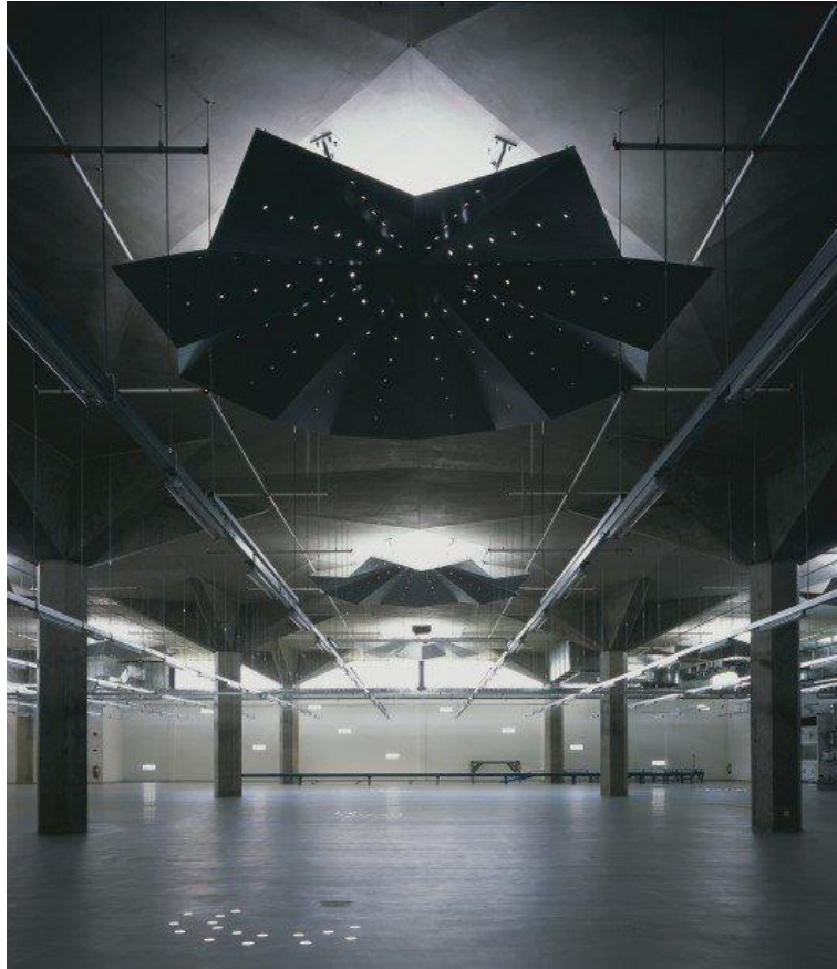
Figure 20: Air well inside the factory.
