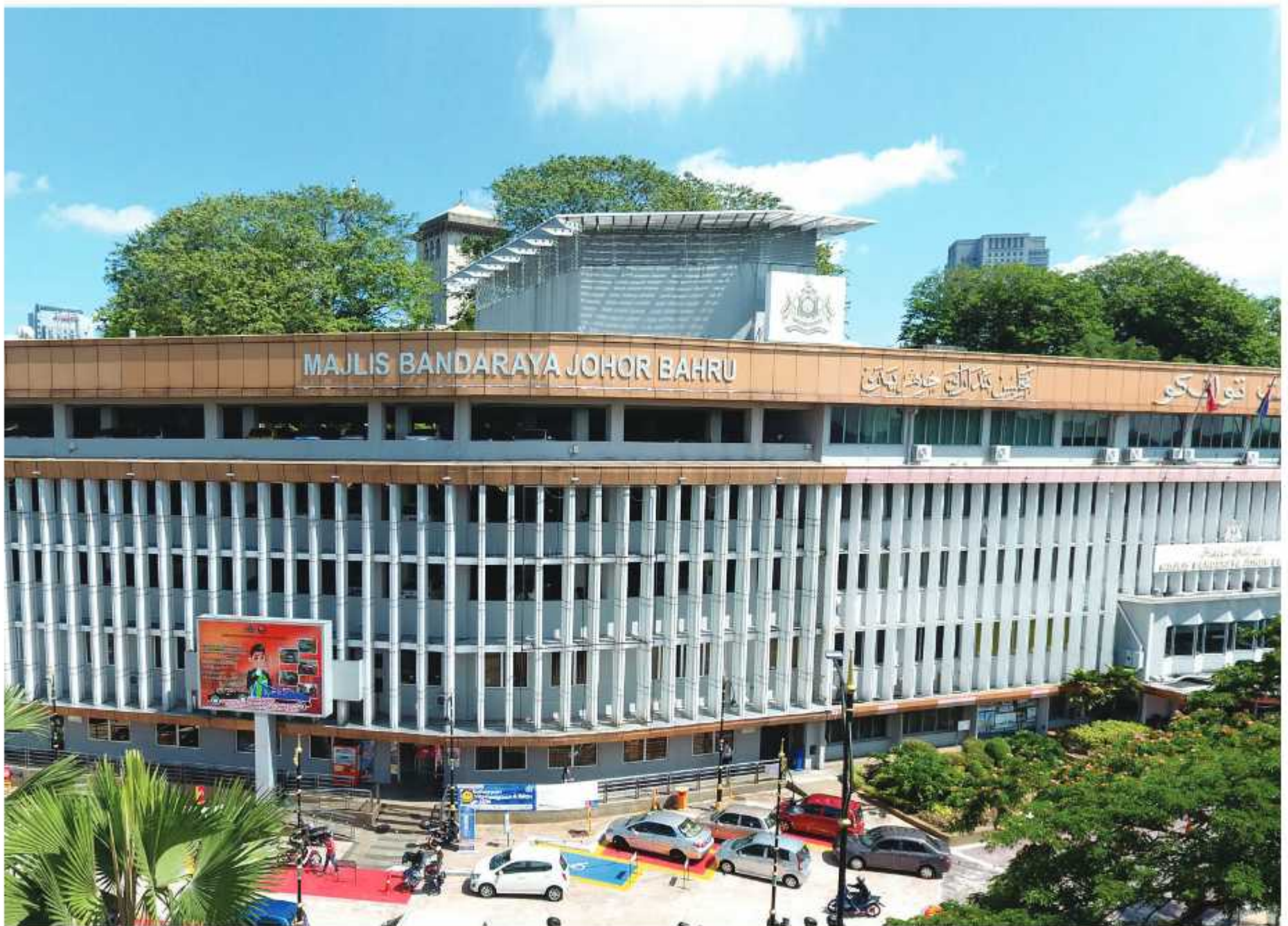
| Pejabat Majlis Bandaraya Johor Bahru The Johor Bahru City Council office.
