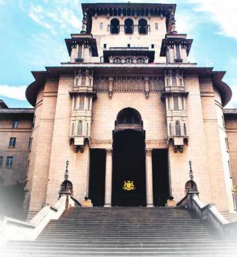
BANGUNAN SULTAN IBRAHIM Sultan Ibrahim Building
