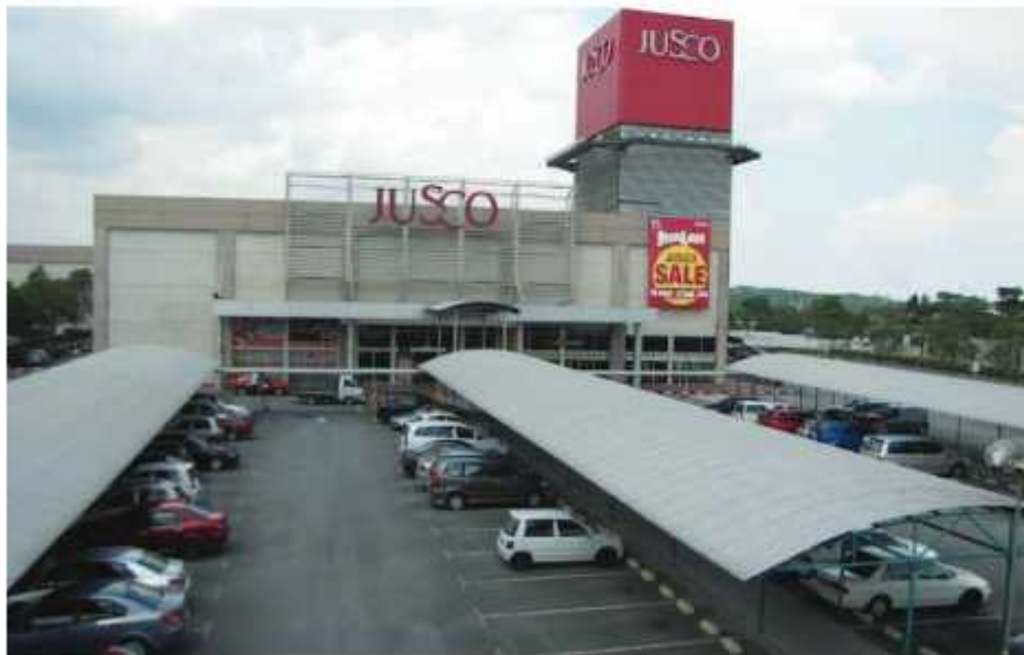
AEON MALL PERMAS JAYA, JOHOR BAHRU
