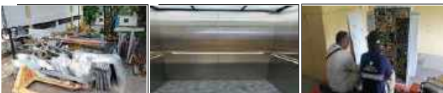
Kerja Pemasangan Lif Plot C Larkin Idaman
