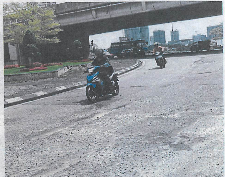
Motorcyclists using this stretch along Jalan Lingkaran Dalam in Johor Baru are dicing with danger as the road is riddled with potholes. - filepic
